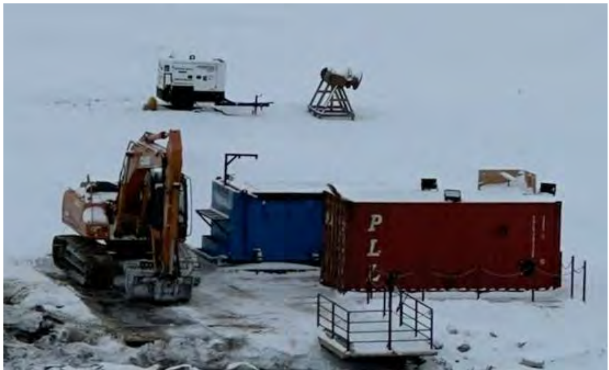
Figure 6: Winter/Spring overview with settling tank installed
