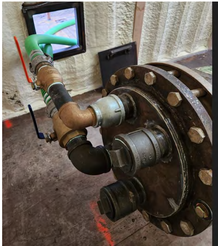
Figure 3: Casing for old intakes with connections installed on custom blind flange
