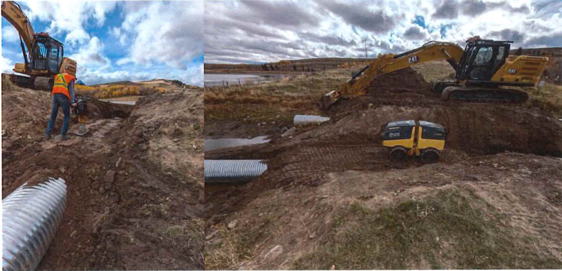
First 4m and 6m sections installed.
