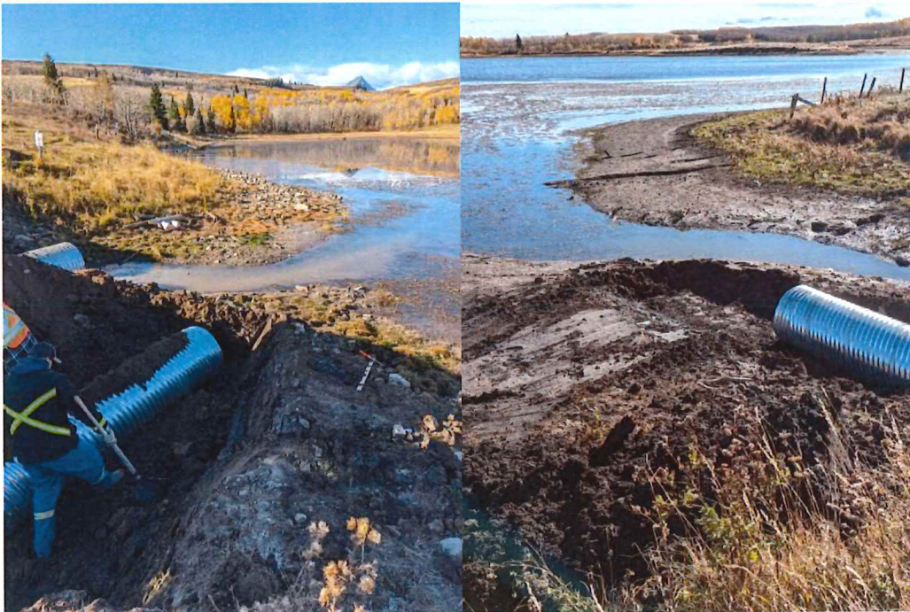
Upper 6m section placed and ready to let upper lake through.
