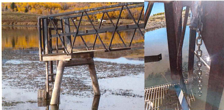
Repair of Gate on dam, to enable lowering of water level.
