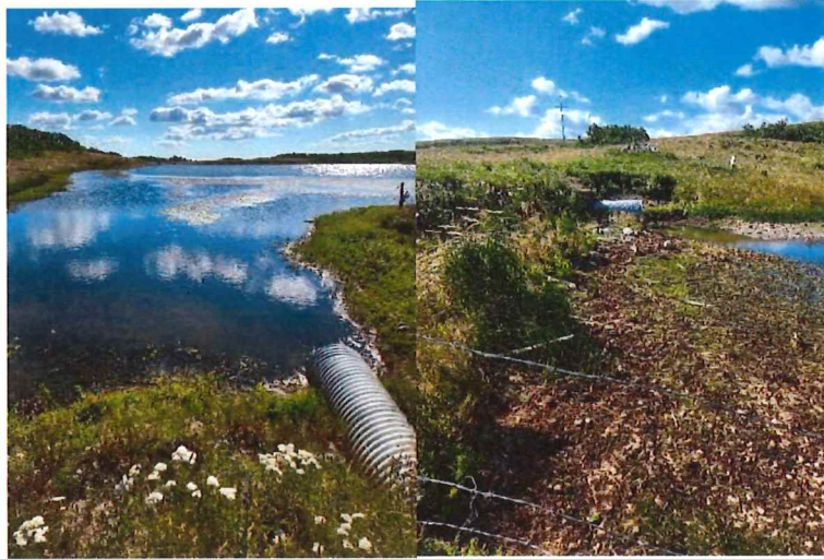
Old existing culvert system between upper lake and lower dam.
