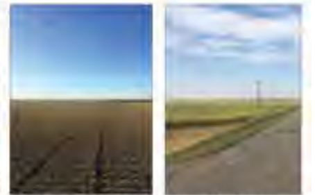
These ruts actually follow a right-of-way between a field that was removed while the ditch to the left of this highway shows extensive encroachment.
